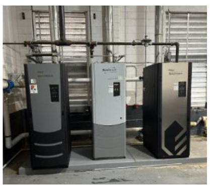
Benchmark Aerco Condensing Boiler with Low NOx Burner
