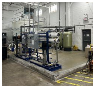
Siemens Vantage M83 Plus Industrial Reverse Osmosis (RO) Water Treatment System
